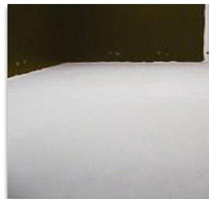
Ready for your finish coat
