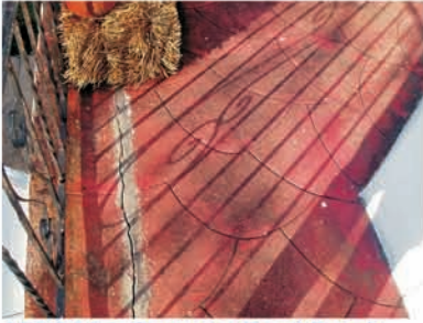
BEFORE - Garage Roof Deck
