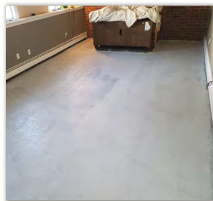
Ready for your finish coat
