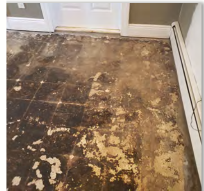
Slab with asbestos adhesive
